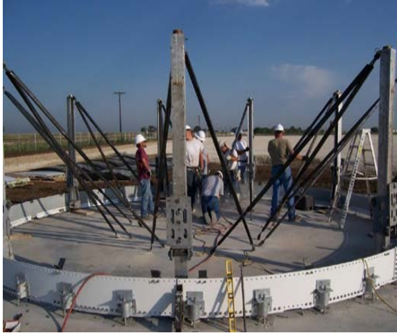
Fig. 2.1 Base construction for tank.
