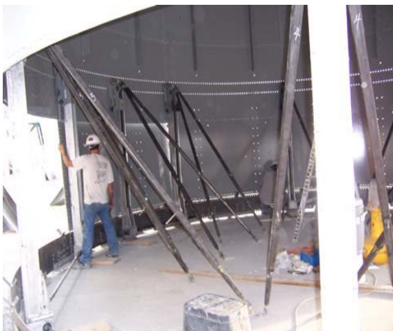
Fig. 2.3 View from inside the tank
