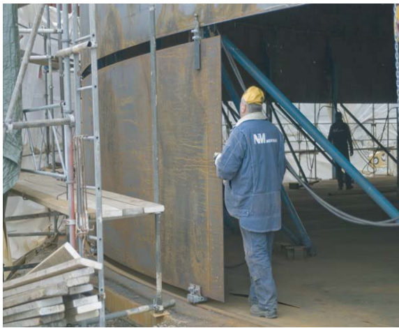
Fig. 2.2 Placing of shell ring sheet
