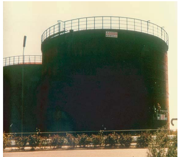
Fig. 2.5 Fully constructed tank
