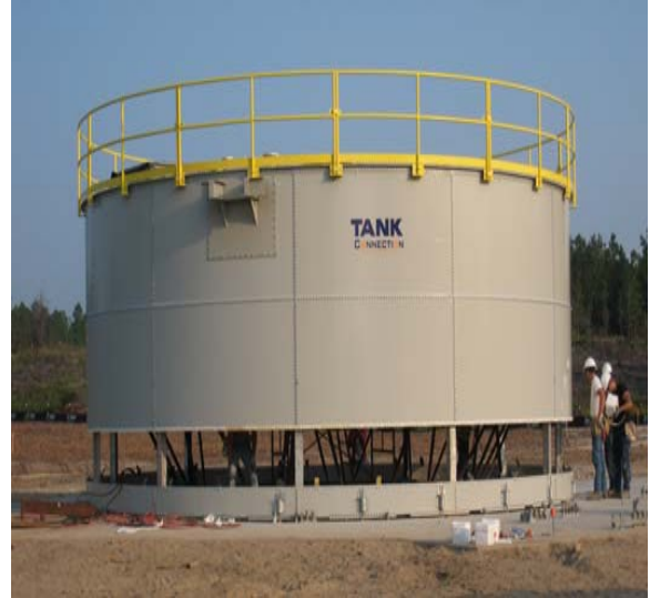
Fig. 2.4 Partial constructed tank
