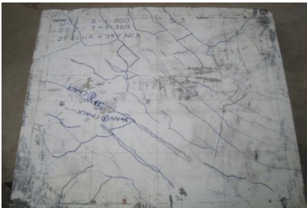
Bottom of slab
