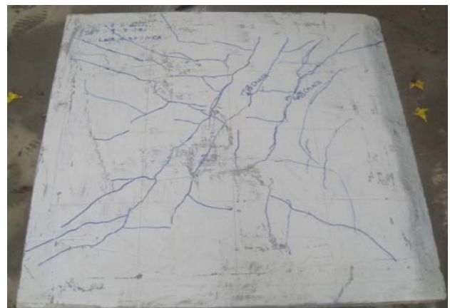
Bottom of slab
