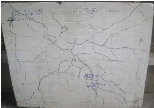
Bottom of slab
