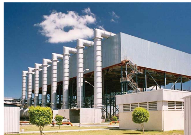
Fig.5. Air Cooled Condenser for a 500MWe Plant
