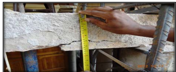
Fig. 4: Measuring depth of flat slab.
